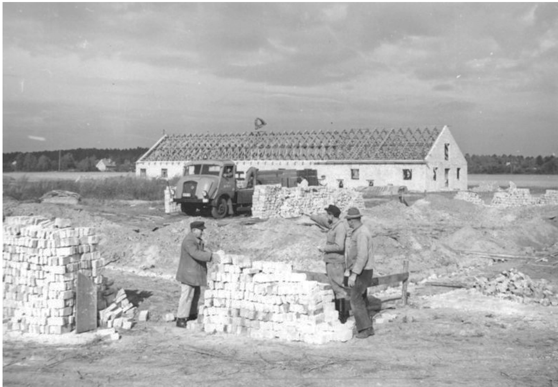
Image 11. The LPG construction brigade builds a feed house on 19 October 1955. Between April and October of that year, the construction brigade completed three new stables. By 1960, the brigade had built farrowing pens, and combines for pigs, cattle, and poultry. All these major construction projects were completed with the help of volunteer construction workers.
