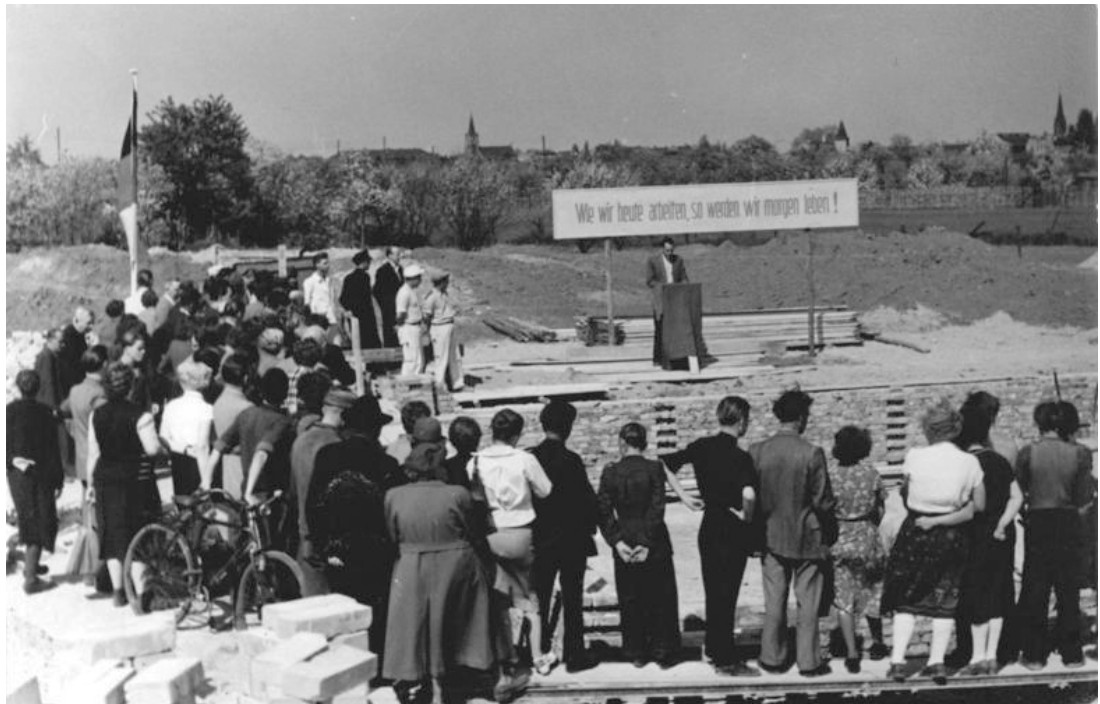
Image 10. On 19 May 1954, the Freie Erde (Free Soil) LPG in Magdeburg-Salbke builds a large farmyard. The cooperative's farmers laid the foundation stone together with workers from neighbouring industrial enterprises. The sign reads: 'How we work today is how we will live tomorrow!'
