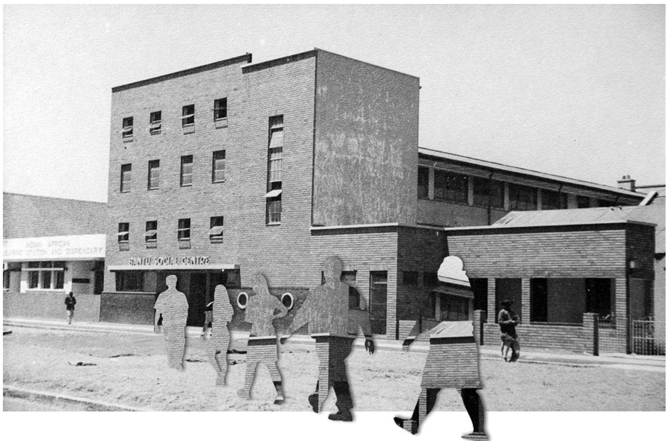
The Bantu Social Centre (now Beatrice Street YMCA) at 29 Beatrice Street in Durban, 1953. Source: Durban Local History Museums
