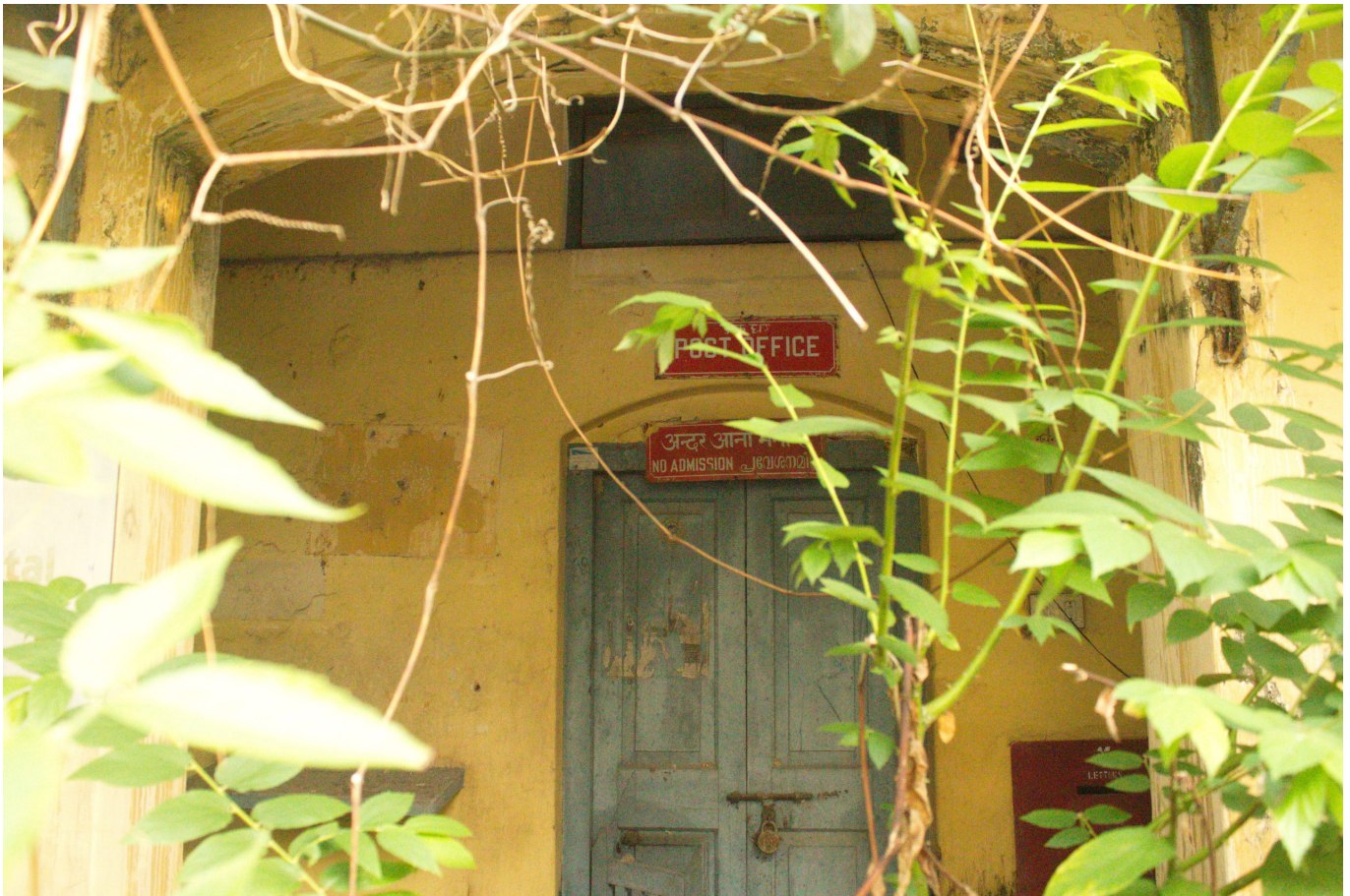
The old Post Office at Mattancherry. There were bullet marks on the walls of the post office as well.
